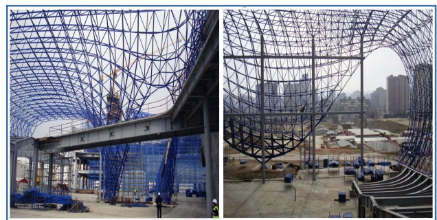
Figure 14: The canopy of steel space frame with double curved freeform geometry and triangular modules [22]
