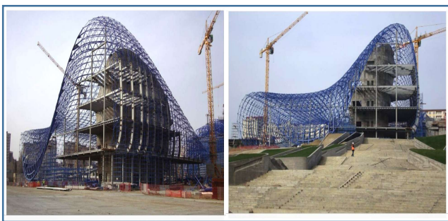
Figure 13: The construction of the centre illustrates the three different structural systems [22]
