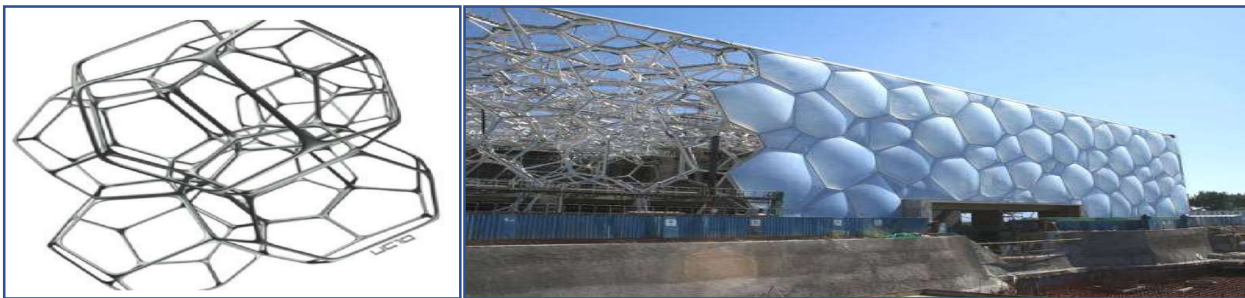
Figure 2: (Left) Weaire-Phelan foam structure. (Right) “Water-Cube” Beijing National Aquatics Centre [18][21]
